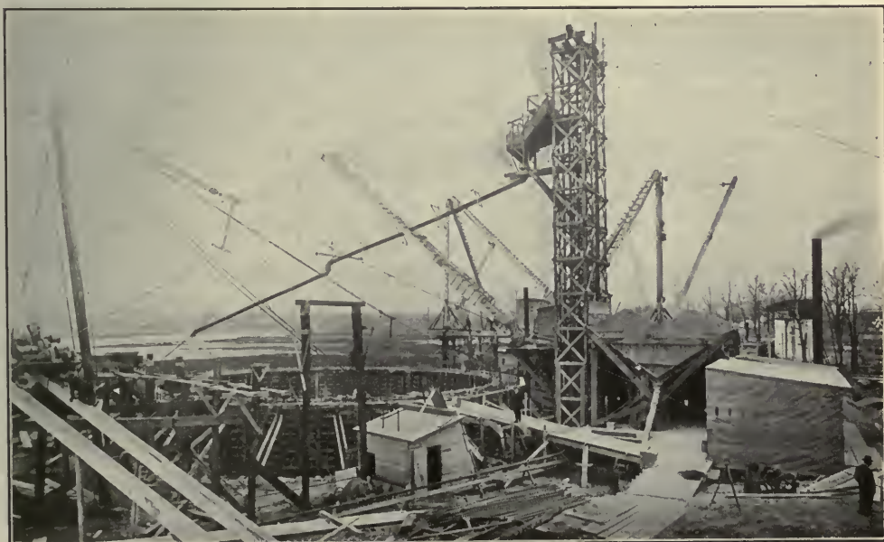
A CONSTRUCTION VIEW, SHOWING METHOD OF POURING CONCRETE FOR CIRCULAR FOUNDATION
